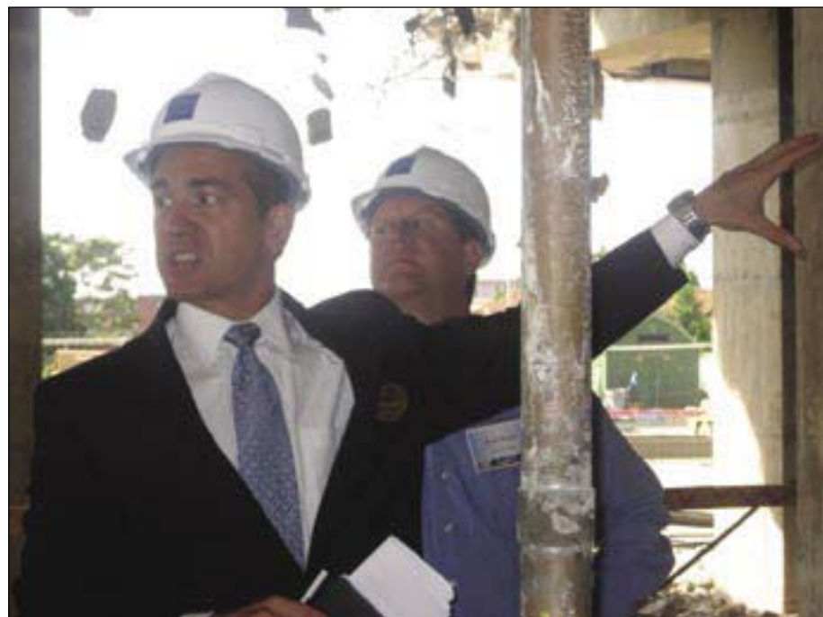
Frank Passanante, regional director of sales and marketing for Hilton Hotels Corp., gestures as he leads a media tour of the renovation project under way at the Hilton Washington. Behind him are the beginning of a new outdoor deck, which is also the roof of a large new meeting space.
